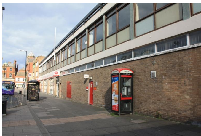
Photograph 3—Keppel Street Post Office to be demolished showing modern brick construction
