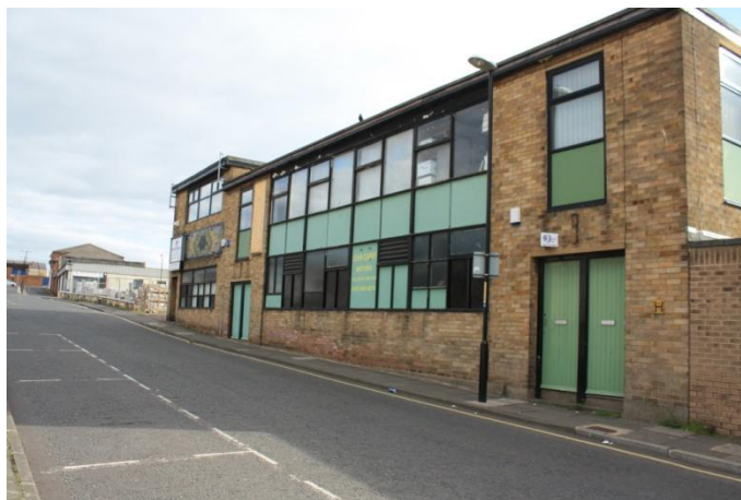
Photograph 2—Buildings on William Street to be demolished showing modern brick construction
