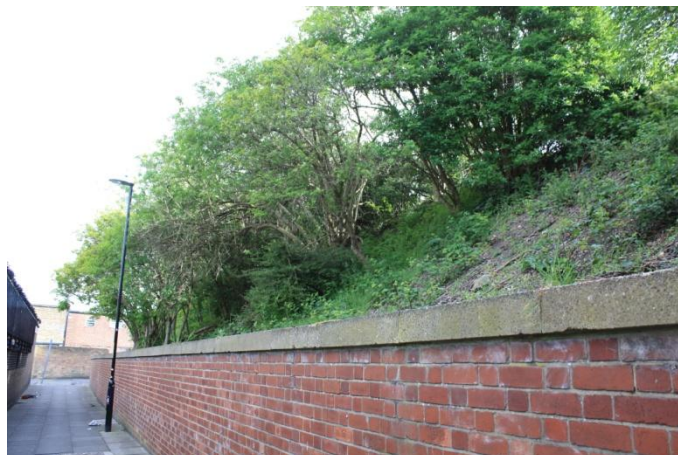
Photograph 1—Scrub on steep railway embankments
